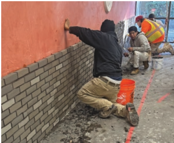
Local 300 Plasterer Apprentices perform EIFS Brick at the local union office.
