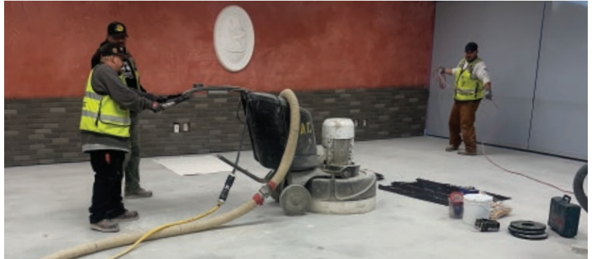
Skilled in their craft local members perform concrete polishing at the local office.
